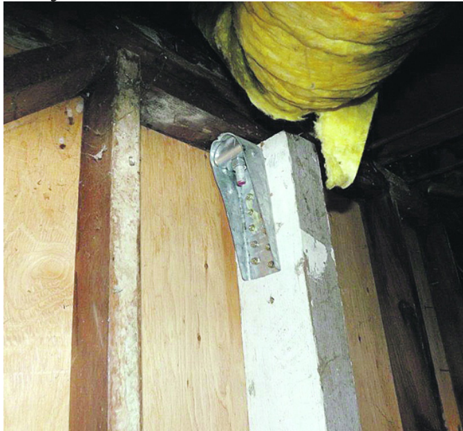
Retrofit bracing Photos Cathy Dausman
