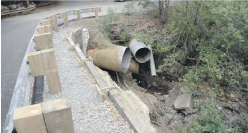
Repairs to an El Toyonal roadside drainage ditch have been added to the City of Orinda's updated Capital Improvement Plan for 2012-2013. Note the aging corrugated metal pipe (CMP). Estimated price tag: \$30,000. Photo provided
