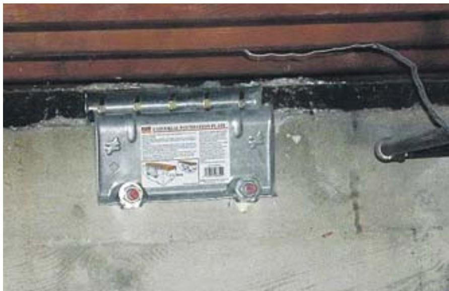
*Foundation plate brace, connects concrete foundation to mud sill*
