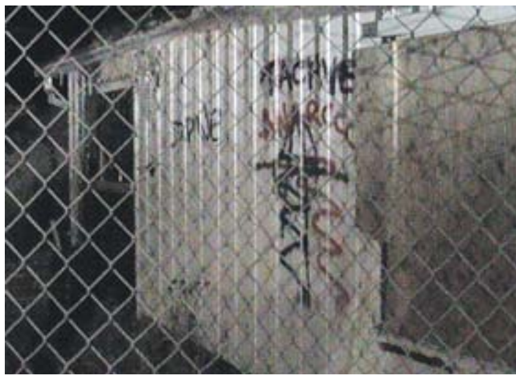
The Moraga Adobe emerges out of the hillside's inky gloom when two Orinda Police officers train their spotlights and flashlights on the structure. Photo Laurie Snyder
