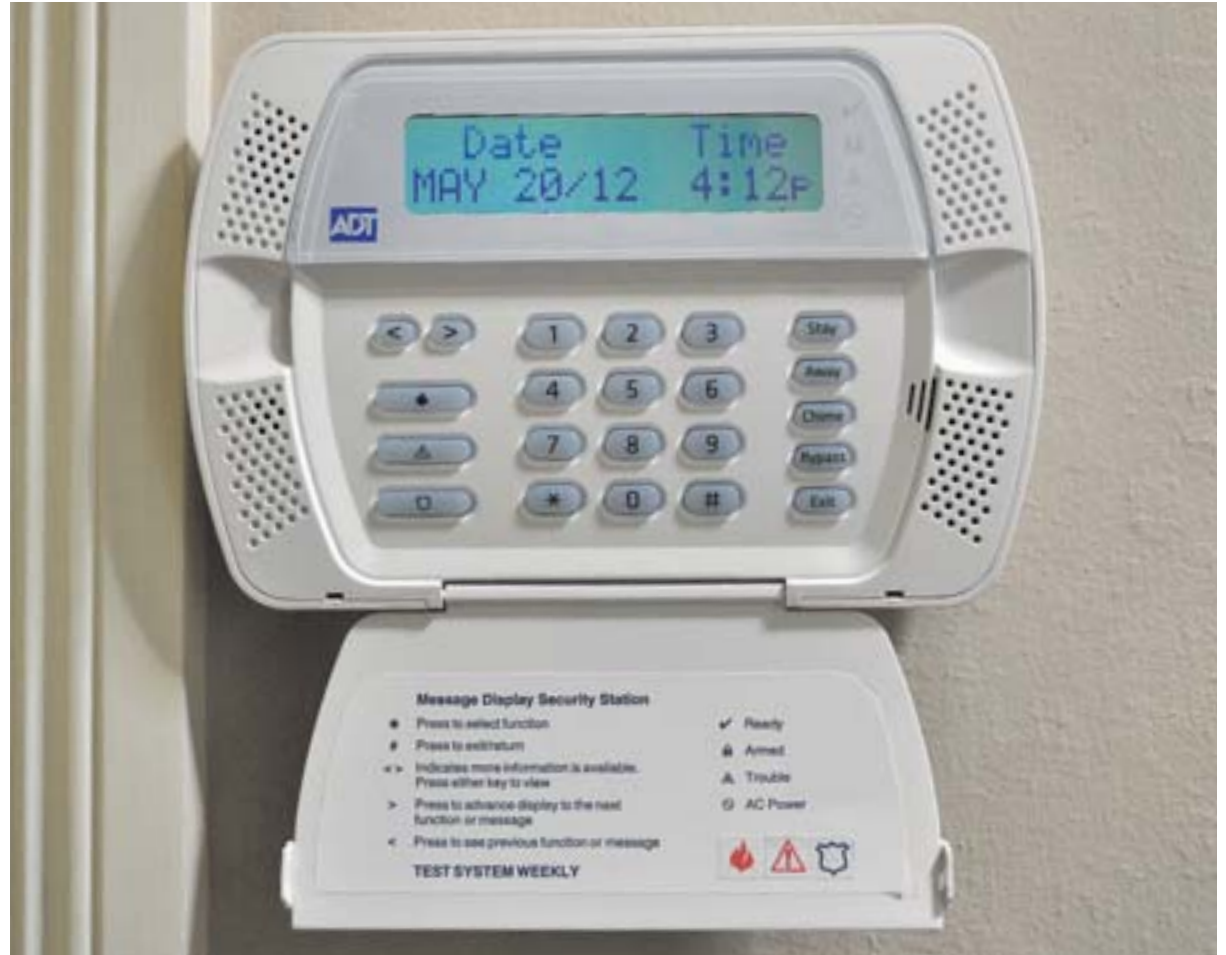
Typical security system control panel
