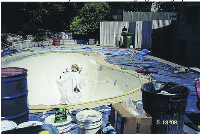
Peter and Nancy Bennett of Moraga resurfaced their backyard pool with fiberglass nine years ago.
