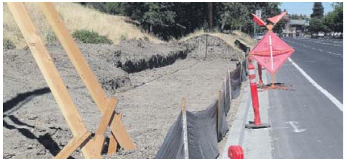
Construction site along Mt. Diablo Blvd.
