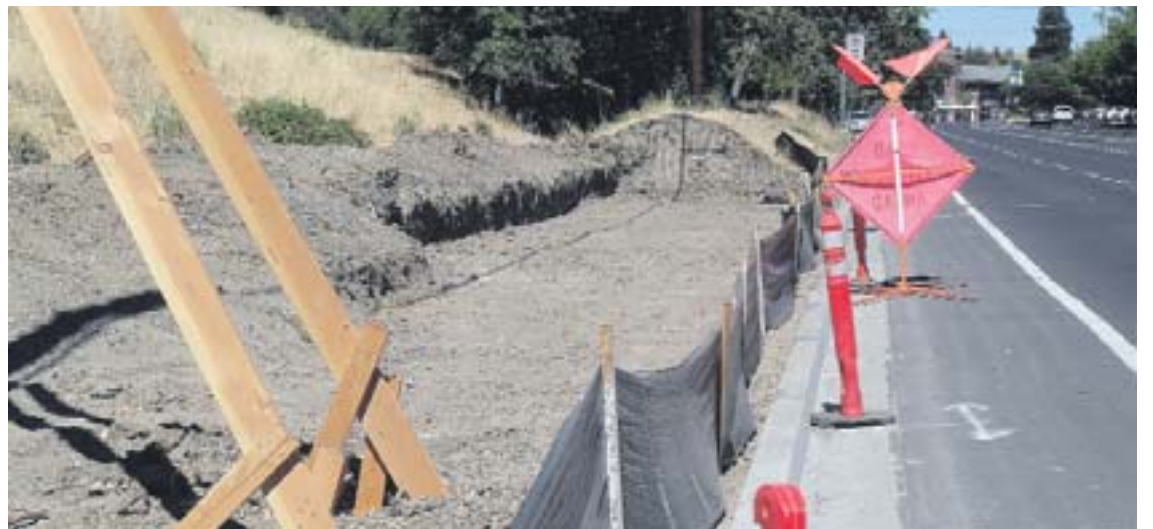
Construction site along Mt. Diablo Blvd.
