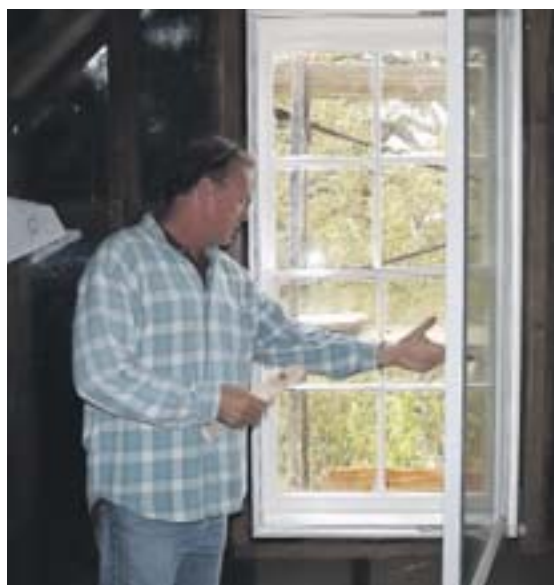
“Triple” thick windows -- dual hung interior windows (new) and a replacement of the original single pane glass outside will give the equivalent of triple hung windows for sound abatement and temperature control.
