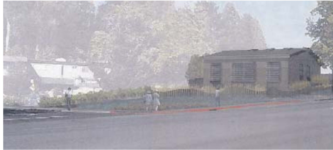
Proposed pumping plant at the corner of Mt. Diablo Blvd. and Mt. Diablo Court
