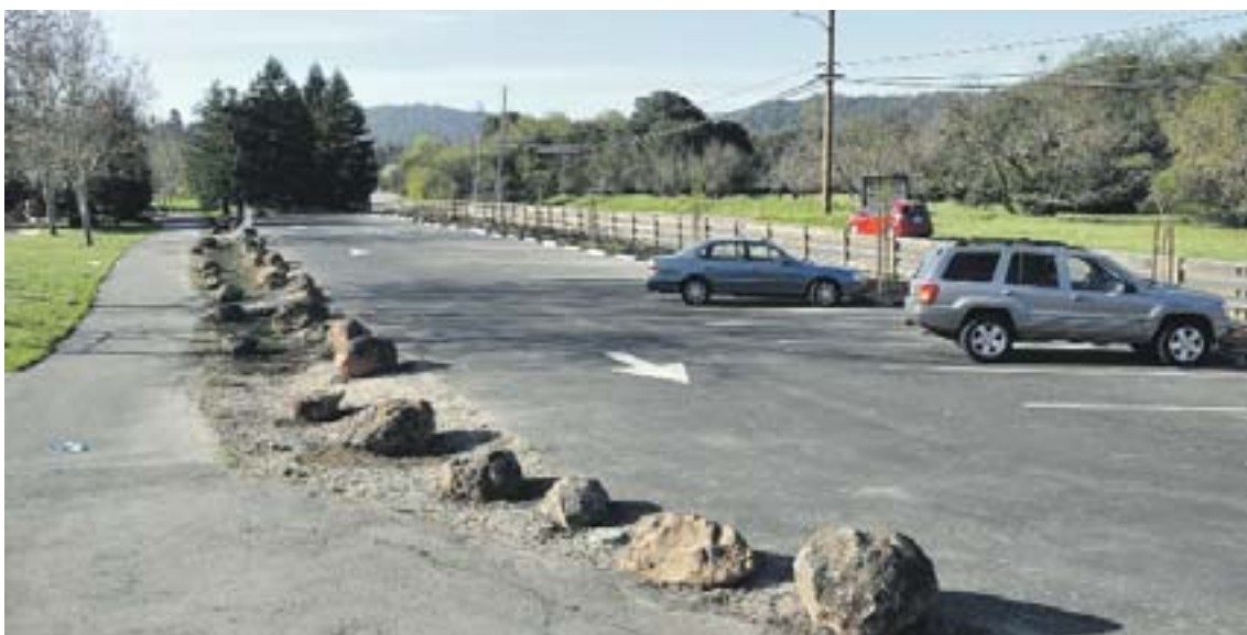
The new skatepark parking lot recently opened on Moraga Road.
