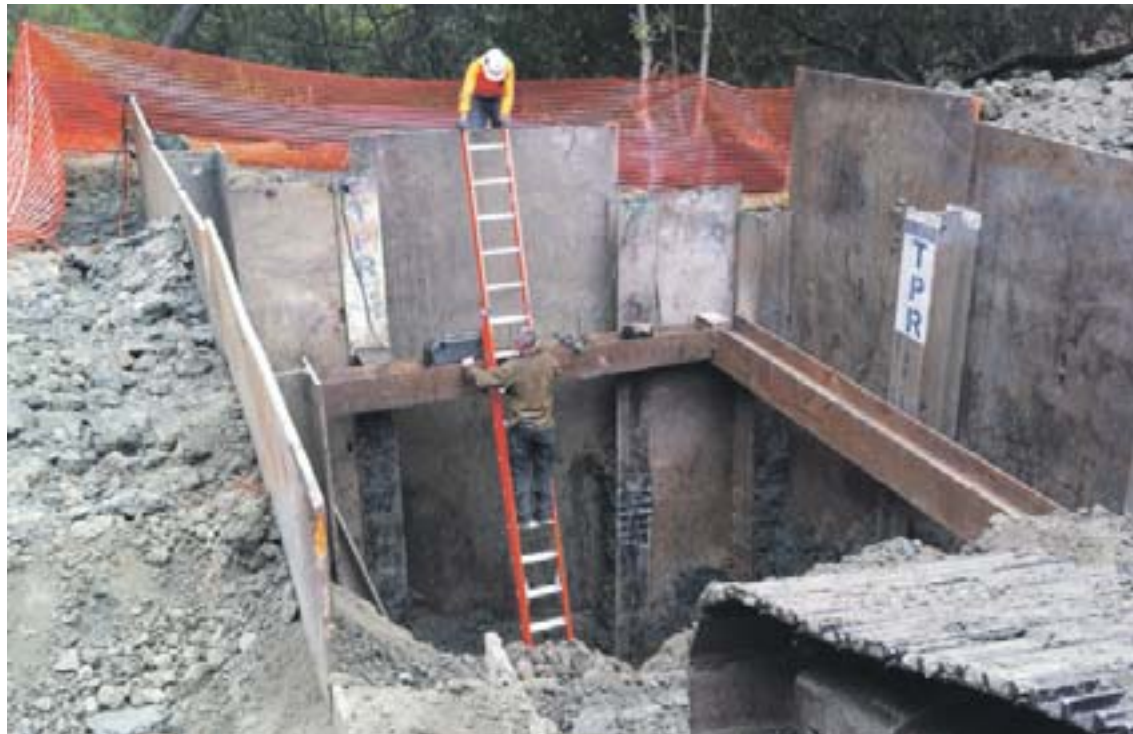
A repair crew is now working its way down to fix a failed drainage system in the Tarabrook neighborhood, which spawned a massive sinkhole last December. A new, sturdier 36-inch concrete drainage pipe will be lowered into this jacking and boring pit—a challenging 25 feet below ground—before workers tunnel and inch the pipe to its final destination. Photo Chuck Swanson
