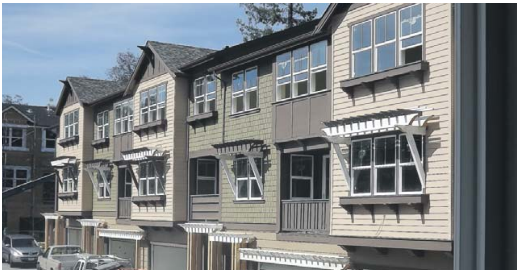
Construction of the Marquis Lafayette development is nearing completion; pictured is a courtside view.
