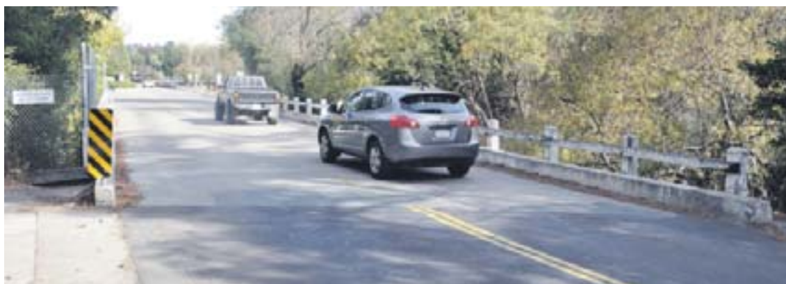
Canyon Road bridge
