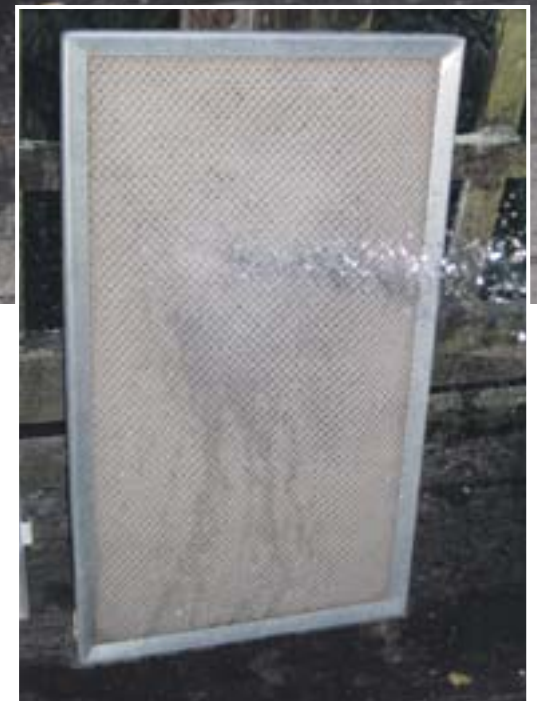
These permanent furnace filters can be rinsed down with a hose – no need to buy new filters.
