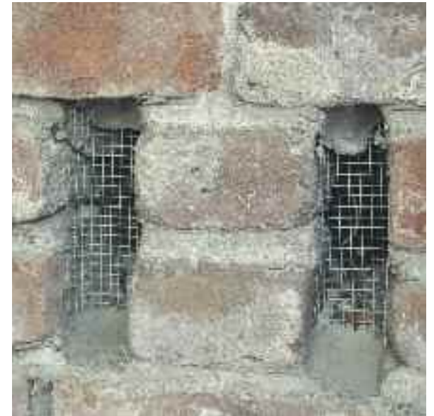
Using 1/8-inch mesh metal screens under eaves or at foundation vents can prevent burning embers from entering a home. Photo Andy Scheck
