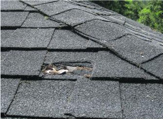
A summer roof inspection can reveal surprises. This hole in a Canyon roof was discovered after a tree contractor left. Evidently a heavy branch pierced the roof, which can lead to problems in the winter rains.
