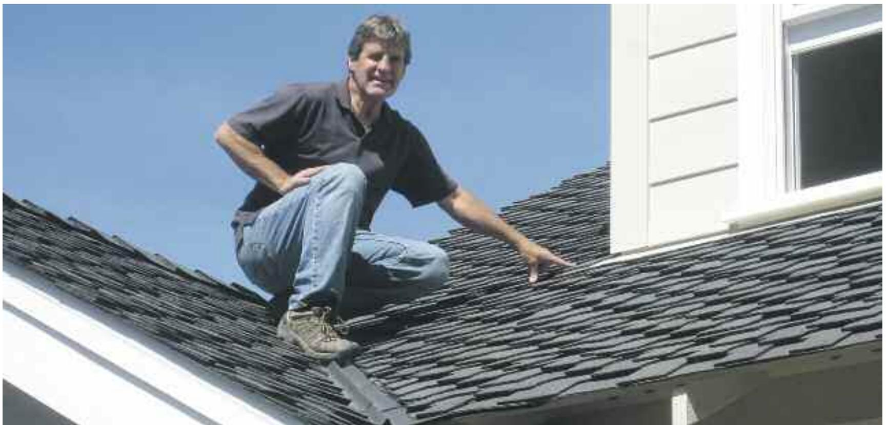
*Roofing contractor Peter Eva of Lafayette points out where summer inspections could begin: where the shingles meet the flashing. Make sure it's overlapping, that there are no gaps, and that debris is cleared.*
