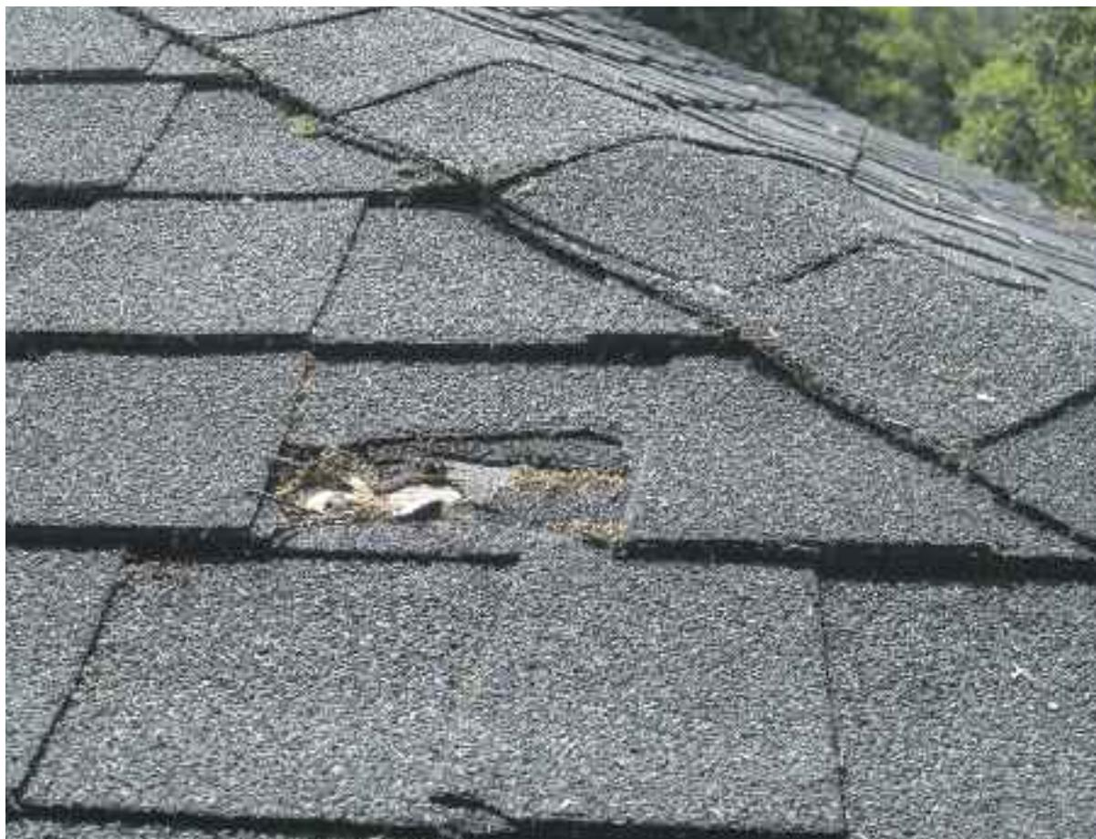
*A summer roof inspection can reveal surprises. This hole in a Canyon roof was discovered after a tree contractor left. Evidently a heavy branch pierced the roof, which can lead to problems in the winter rains.*
