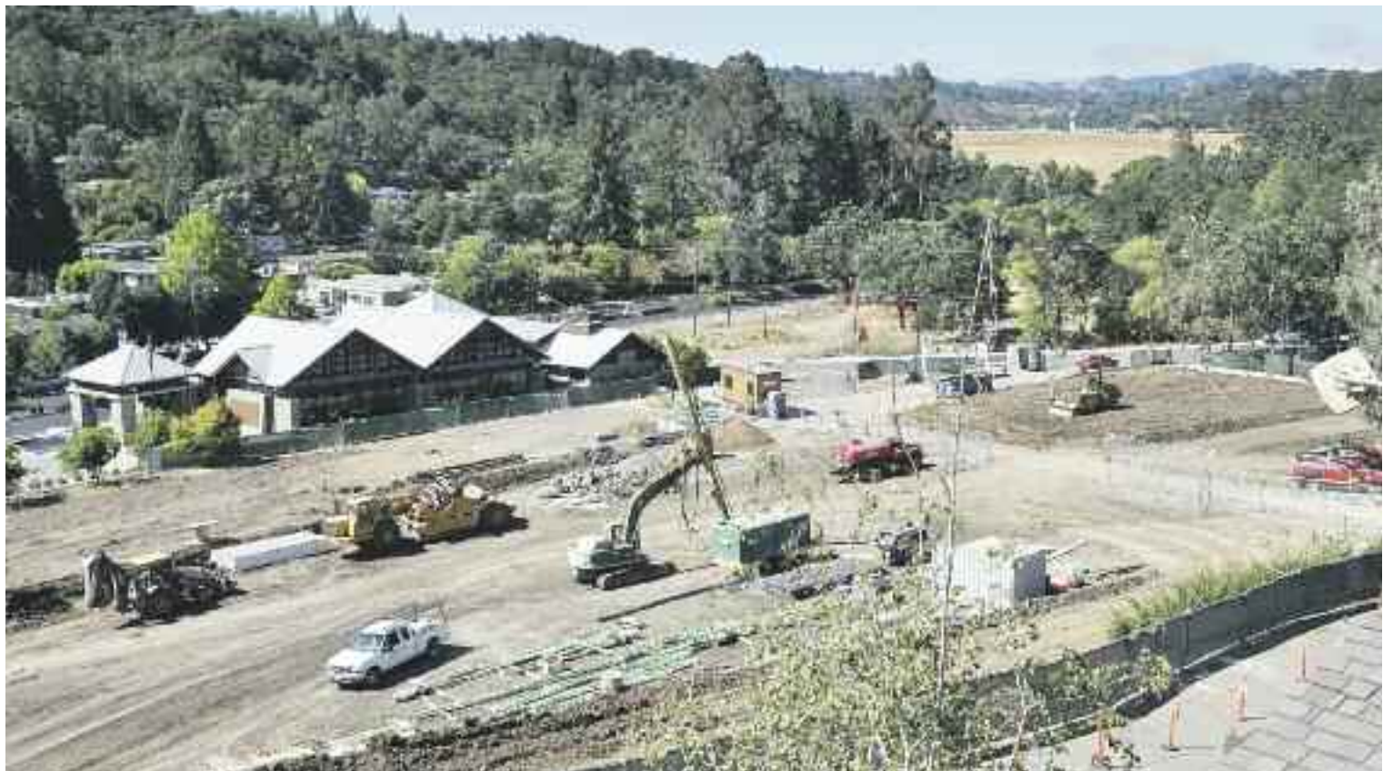
View looking down on the Woodbury construction site.
