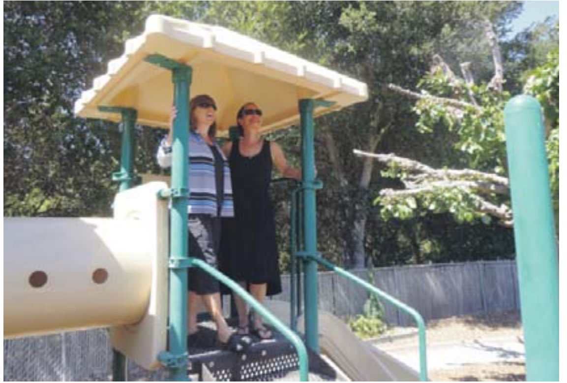
From left: Susie Allison and Cathy Harris climb on a play structure at Mulberry Tree Preschool to take a look at the new roof. Photo Sophie Braccini
