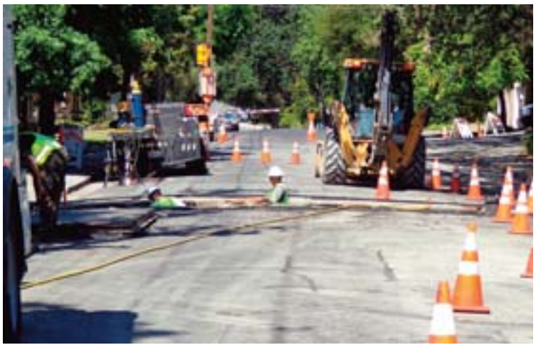
Brook Street is closed near Moraga Road for EBMUD, where workers are replacing over 500 feet of pipe that was installed in 1933. Photo Cathy Tyson
