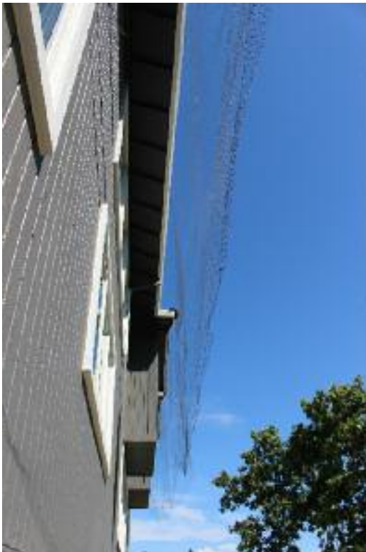
Some houses, such as this one in Orinda, sport bird nets to keep the woodpeckers away from the siding. Photos Chris Lavin
