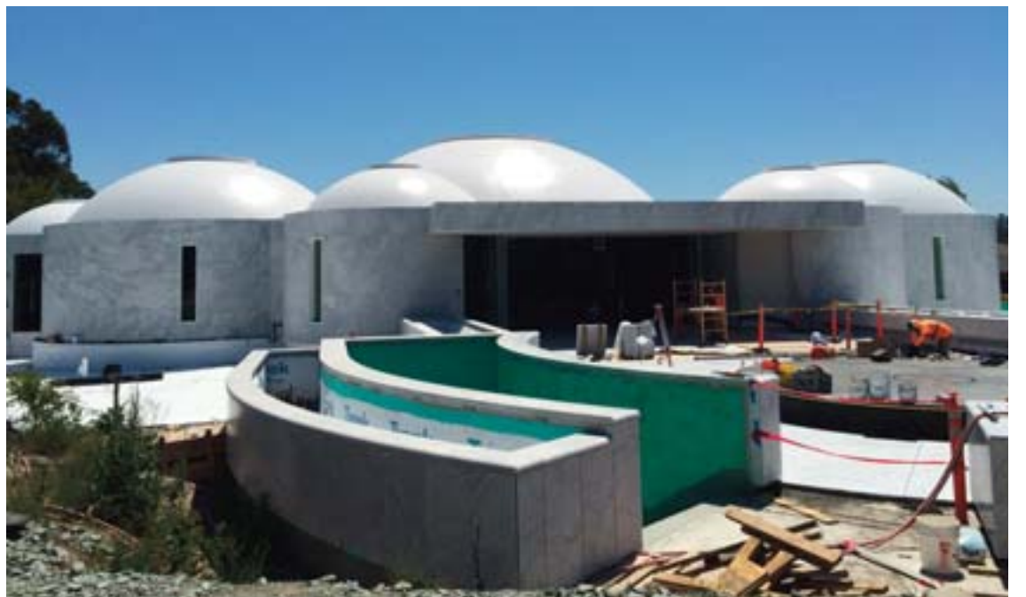
Sufism Reoriented Sanctuary construction site
