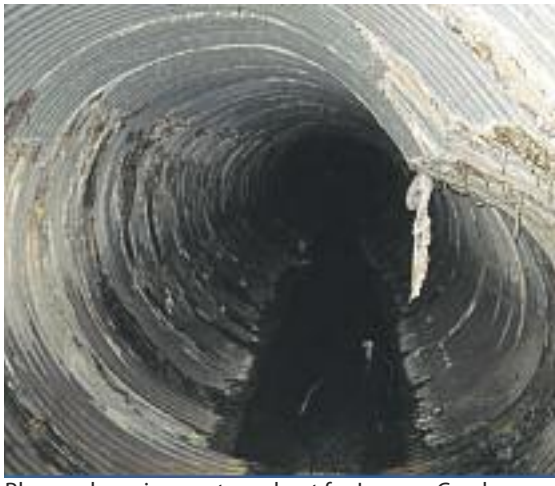
Rheem shopping center culvert for Laguna Creek
