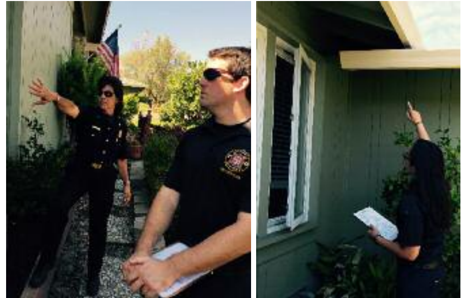
MOFD Fire Marshal Kathy Leonard (left) and MOFD aide Steven Woods evaluate where leaves could collect on a brush proximity to siding at the reporter’s house. MOFD aide Jessica Misleng shows where leaves could collect on a roofline, increasing fire danger. Photos Cathy Dausman
