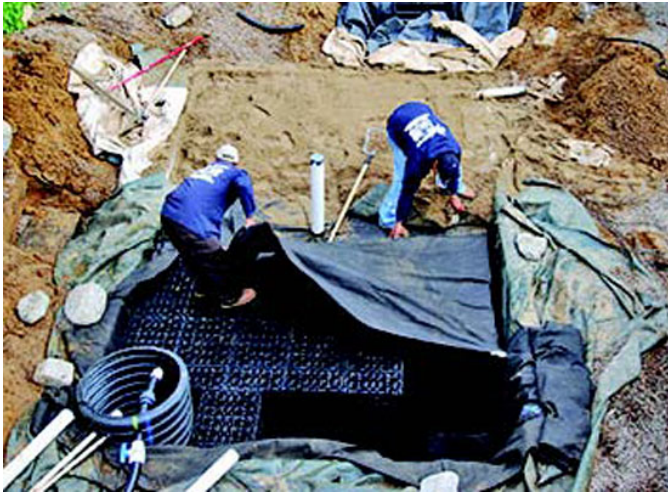
Swimming pool to rain tank conversion Photo provided
