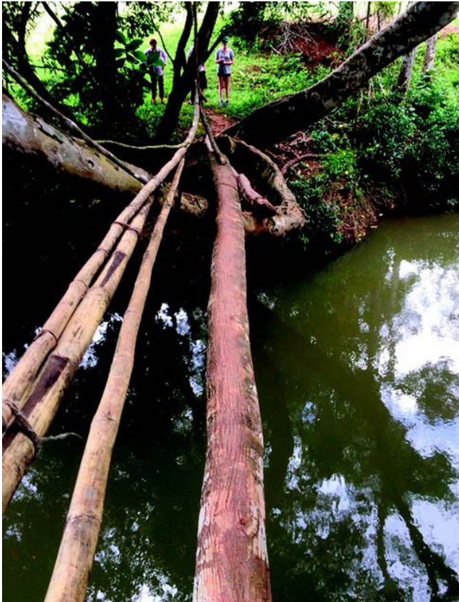
The old bridge was made of branches from trees growing on both sides of the river.
