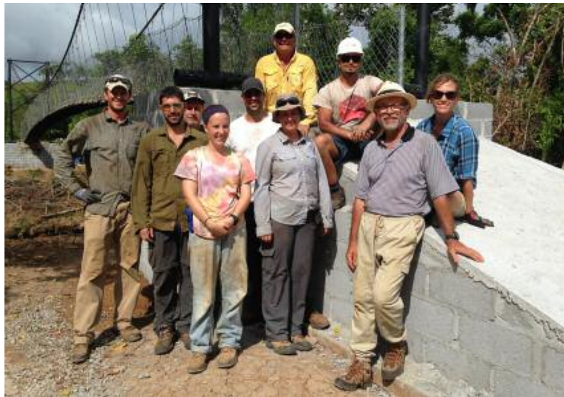
The happy team in front of the finished bridge
