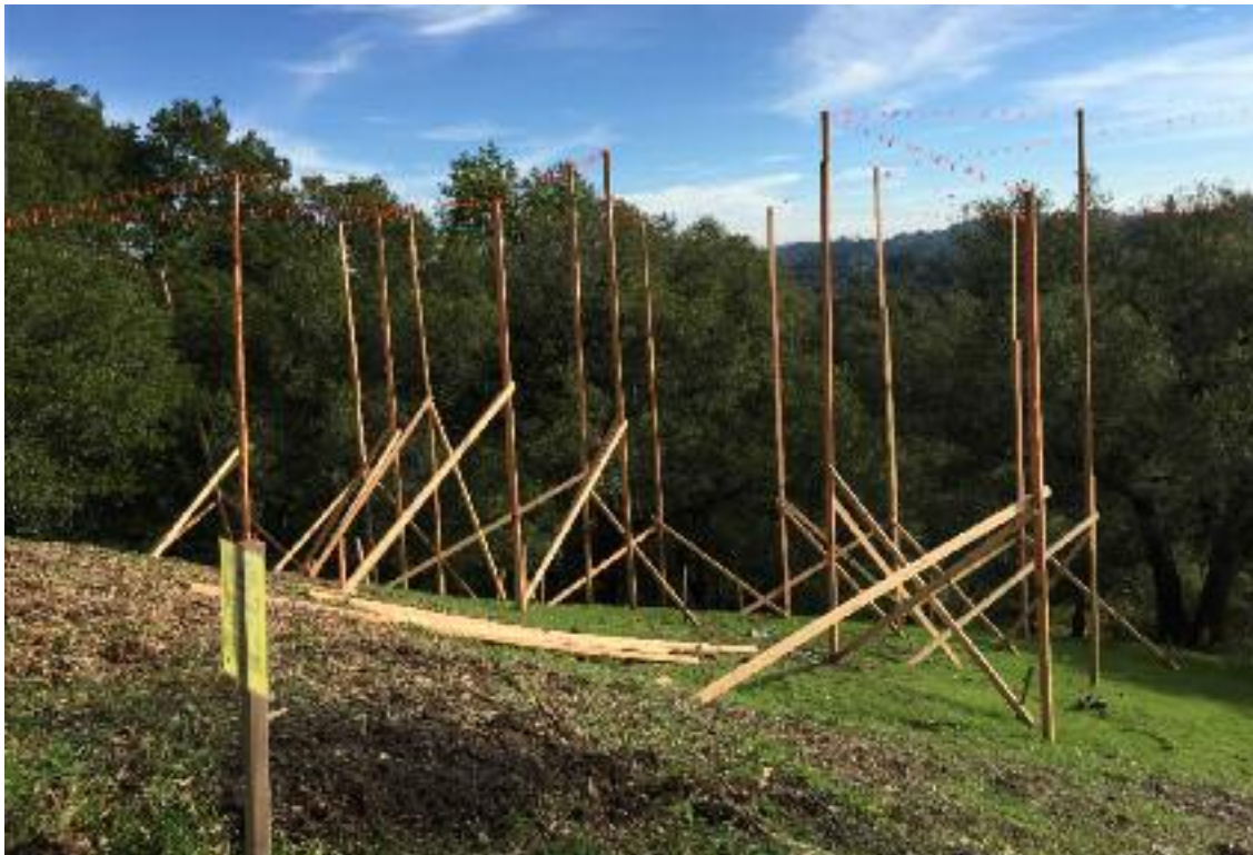
Story poles can help to visualize the impact of the development in an existing neighborhood Photo Cathy Dausman
