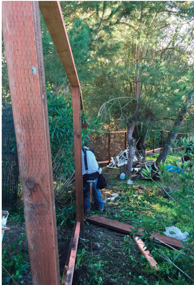
A crew builds a fence. Photos Cynthia Brian
