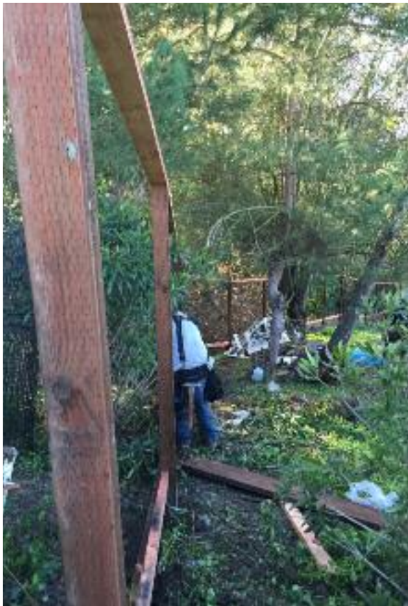
A crew builds a fence.
