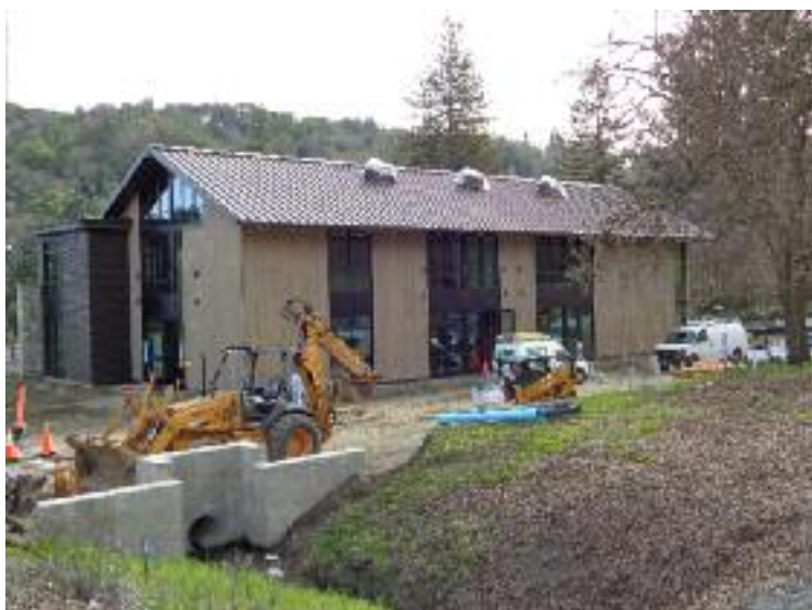
A view of the completed Eco Vive building
