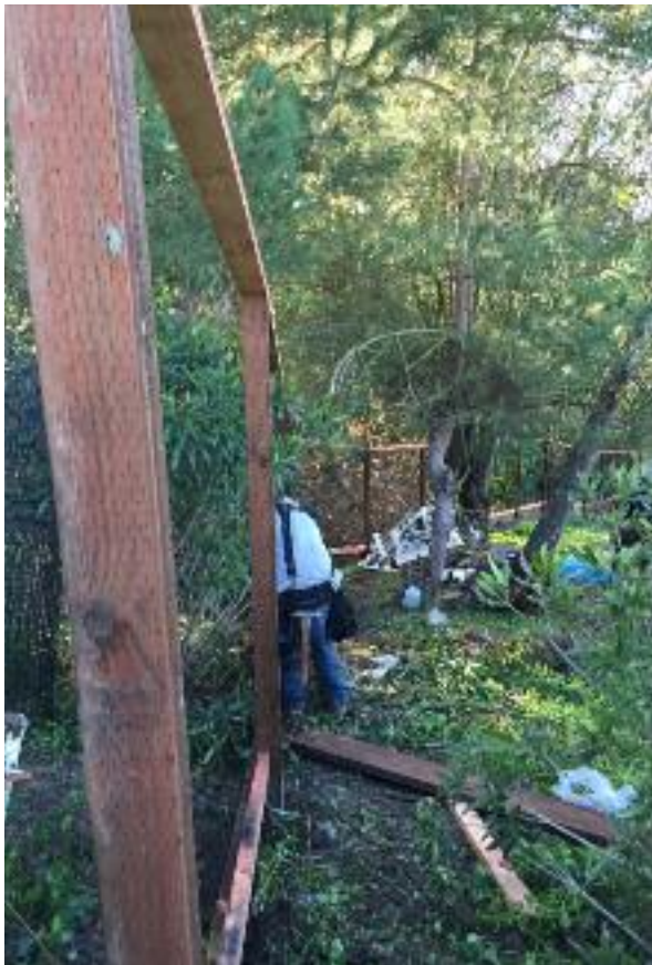
A crew builds a fence.
