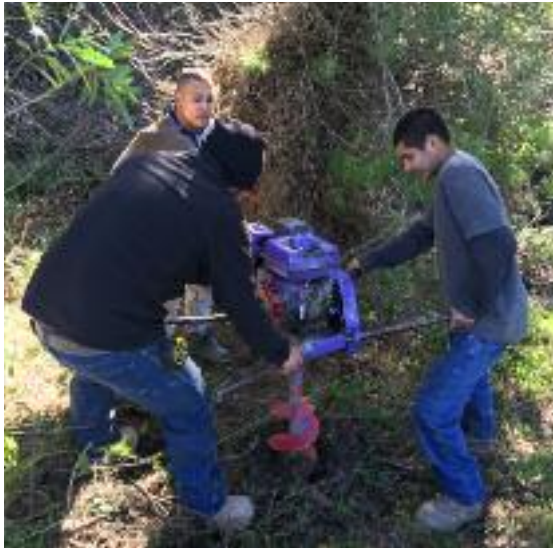
A crew with a post hole digger.
