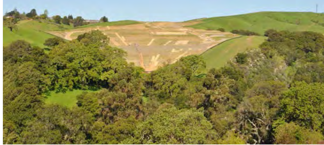
The Bellavista development is under construction off Rheem Blvd.
