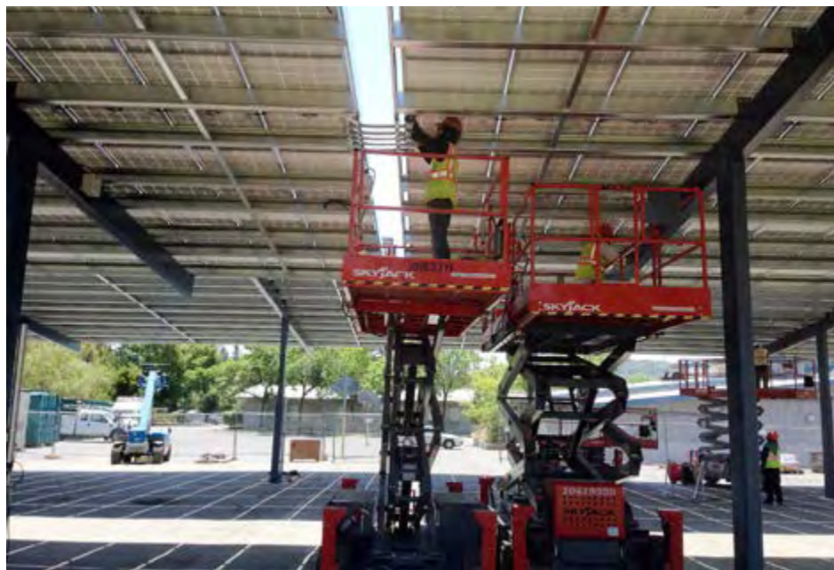
Workers install solar panels at OIS.
