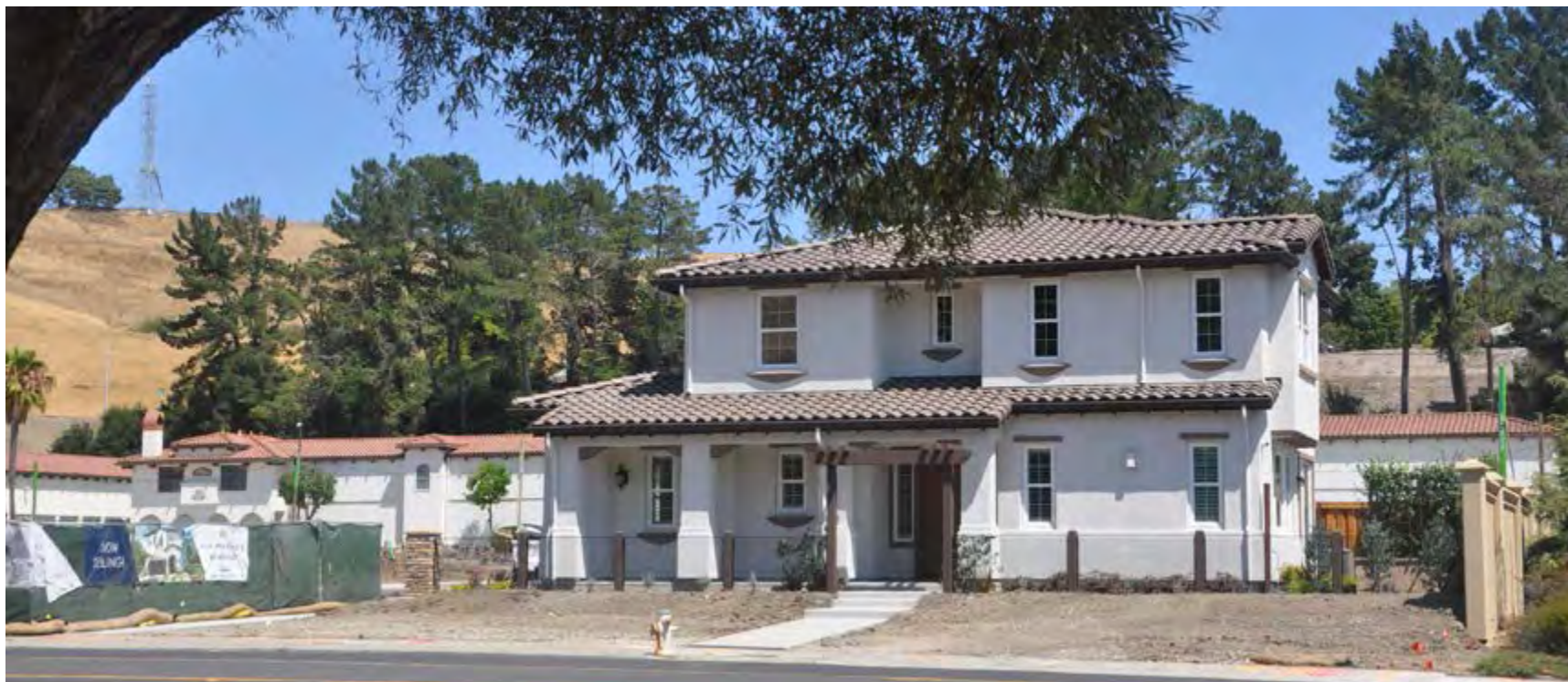
First house in the new development Via Moraga on Moraga Road
