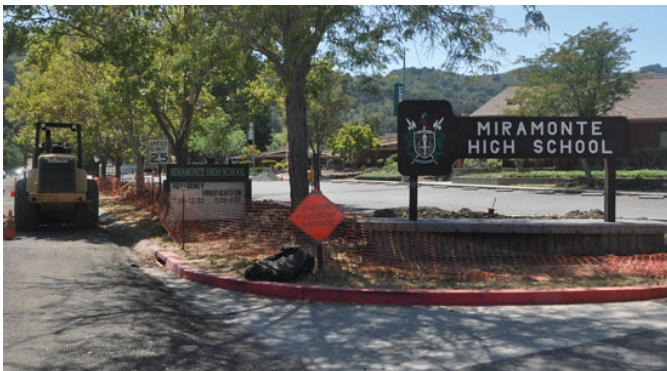
The road, sidewalk and parking lot at Miramonte High School are still under construction. Photo Andy Scheck
