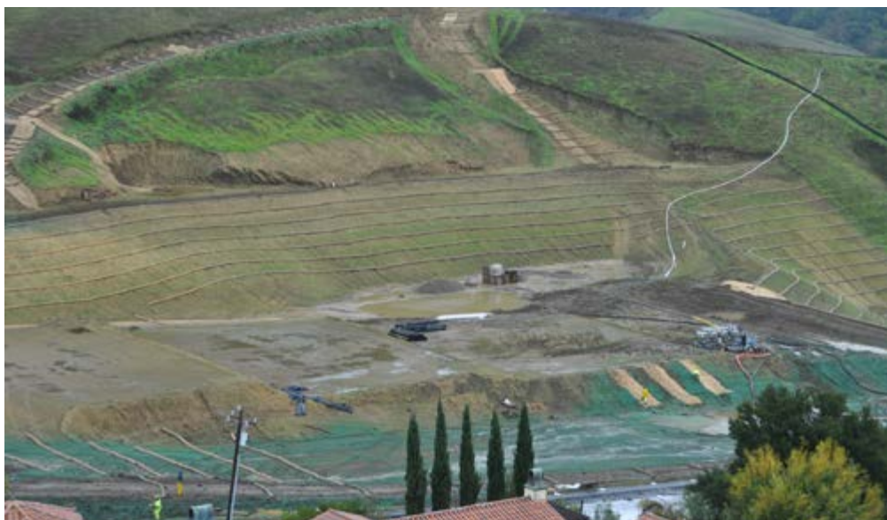
A landslide is slowing work at Bellavista.
