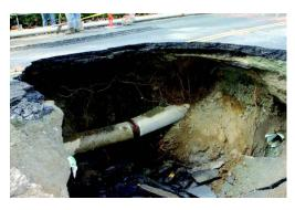
Sinkhole reveals broken culvert that requires a new large diameter pipe to contain major EBMUD water main, PG&E gas pipes, and Contra Costa County Sanitary District sewer pipes. Photo Gint Federas
