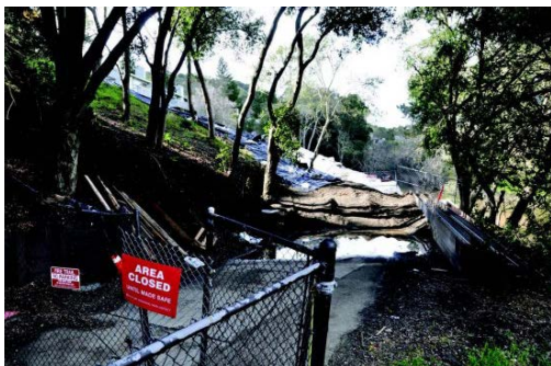
A landslide blocking access to the trail Photo A. Scheck
