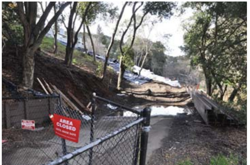
A landslide blocking access to the trail
