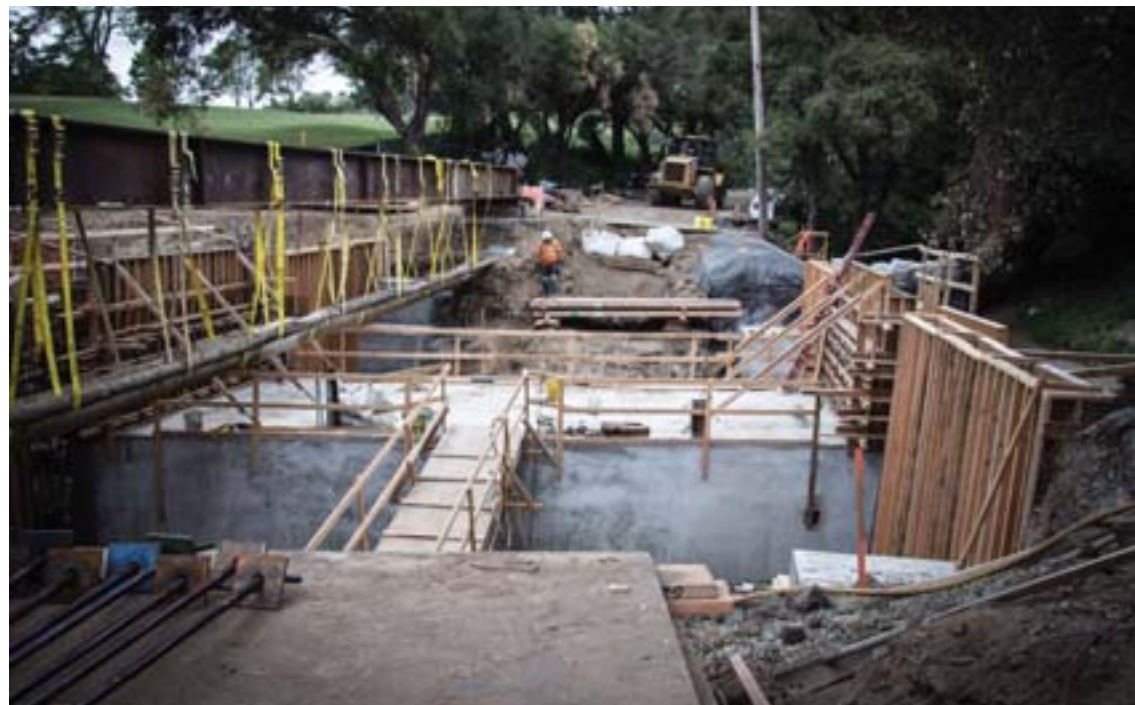
Repair work on the Miner Road sinkhole is progressing nicely.
