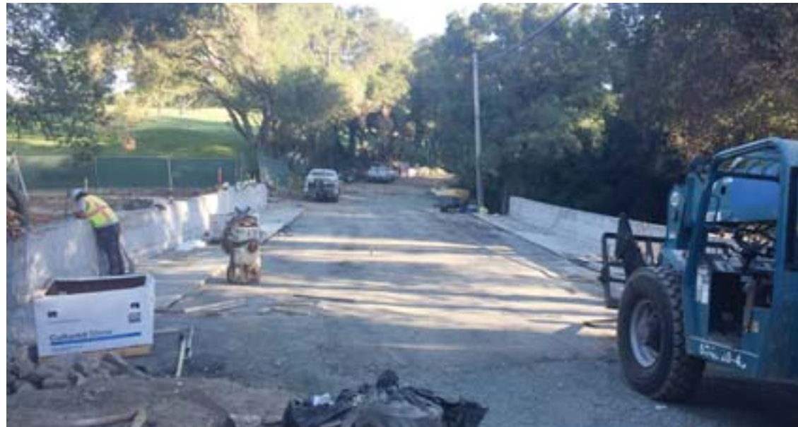
Near completion: Miner Road will be open to traffic on July 3.
