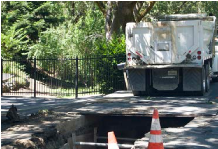
EBMUD installing a new pipeline.
