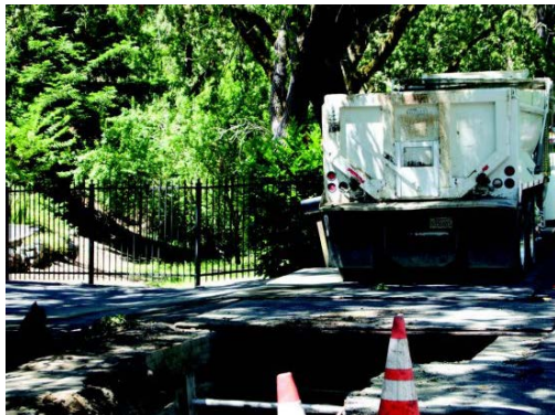
EBMUD installing a new pipeline. Photo Pippa Fisher
