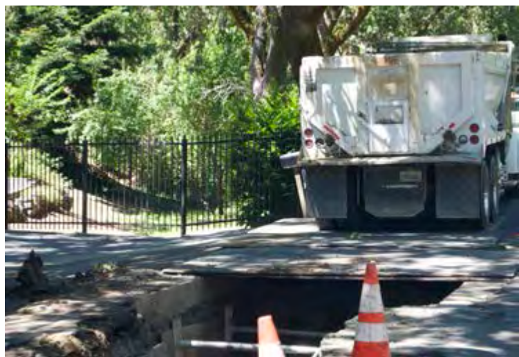
EBMUD installing a new pipeline.
