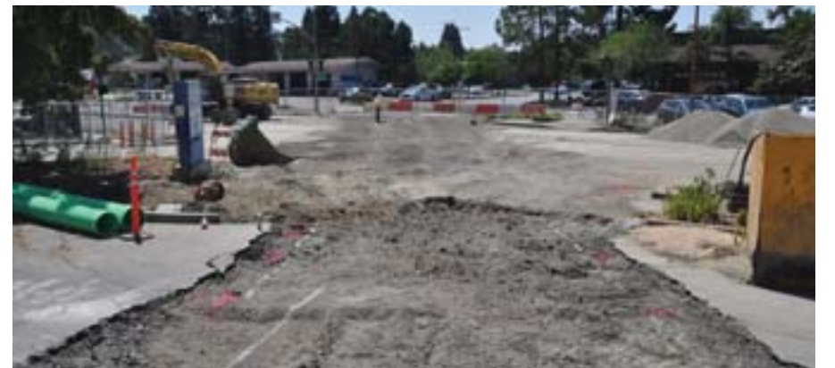
The sinkhole site during construction
