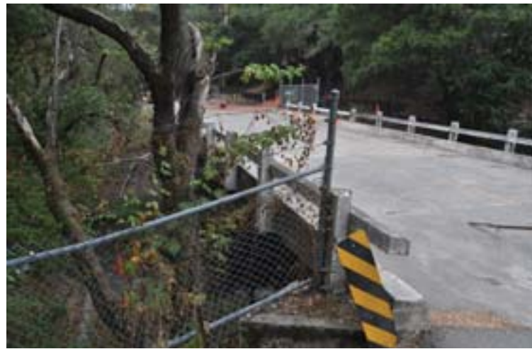
Canyon bridge remains closed
