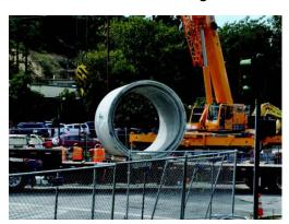
On Sept. 18 WC Maloney Inc. started preparation work for the removal of Canyon Bridge. On Sept. 20 the heavy duty equipment should arrive and demolition will begin. The first two days of the week were used to protect the creek bed so debris is not carried by the current. At the same time installation of the concrete replacement culvert began in the sinkhole. Once this is finished, the sections will be sealed before the hole is closed and the
