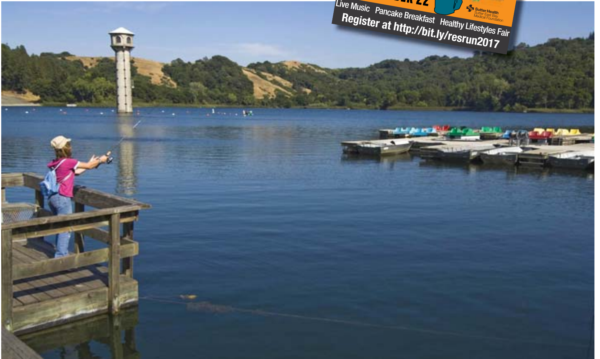
The 90-year old Lafayette Reservoir tower slated for retrofit.
