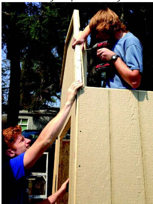
Jackson Reilly at work with friends on the shed. Photo provided
