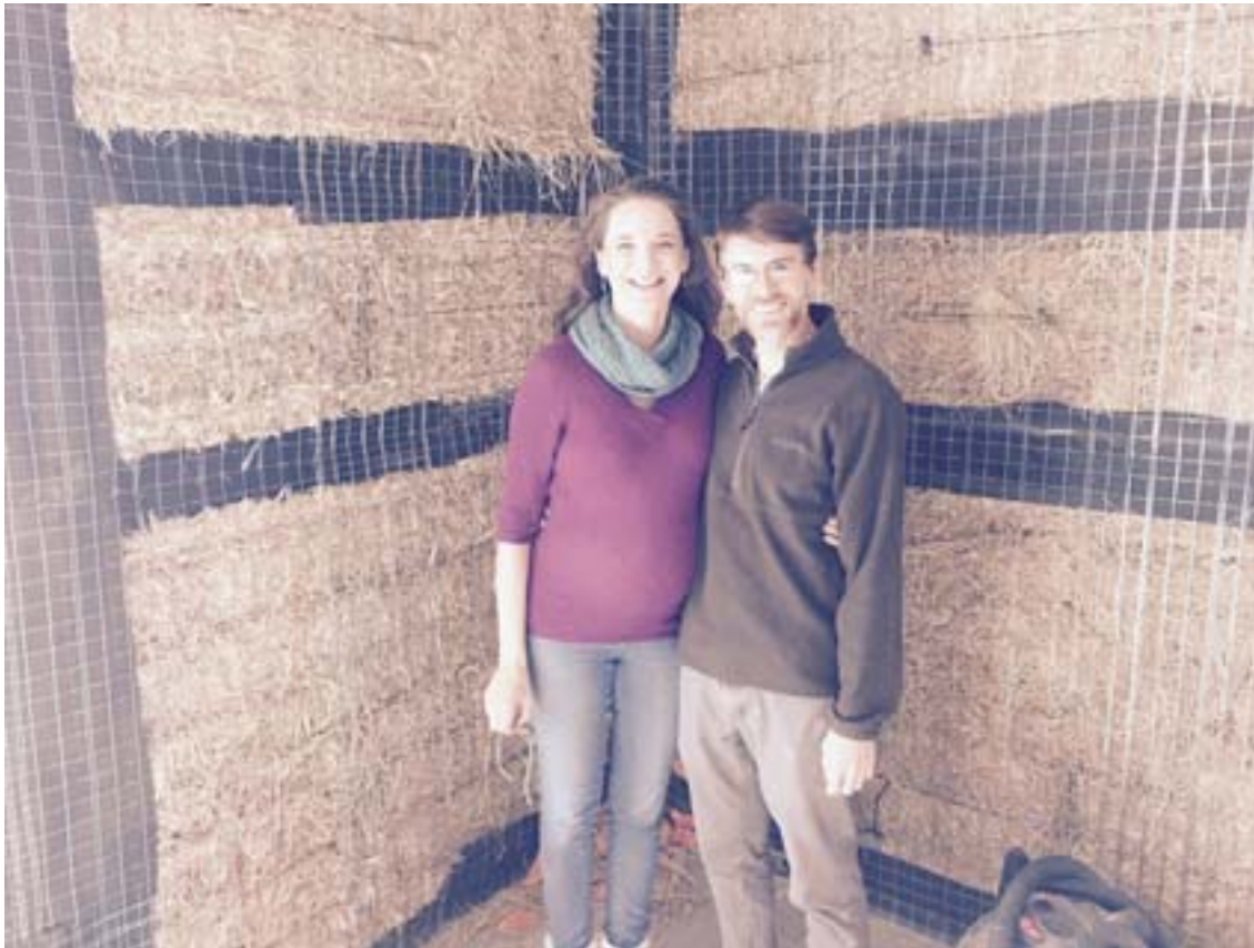
Amber and Norman Remer smile inside their house of straw, while under construction.
